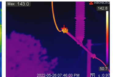
Power Industry Inspection
